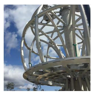
Prior to delivery on-site, several non-destructive tests were conducted to ensure the structural integrity of every element and guarantee the pieces would fit together perfectly. All elements were then protected by hot dipped galvanisation post fabrication and then a three coat paint system, ensuring ultimate longevity of the structure.
